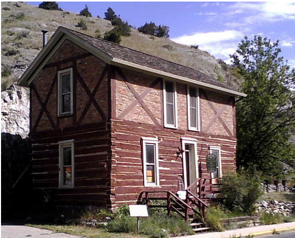
A variation of the second meaning of half-timbered: the ground floor is log and the upper floor is framed (half-timbered in the first sense). Kluge House, Montana, U.S.A. Image: Library of Congress, Prints & Photographs Division, MONT,25-HEL,1-2
