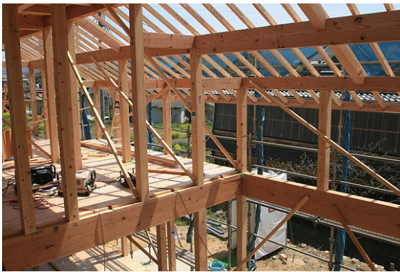
Pin-connected post and beam house framing
