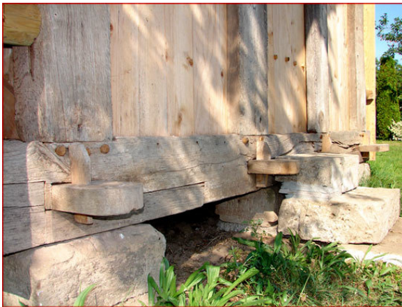
Through-wedged tenons used on a French granary.
