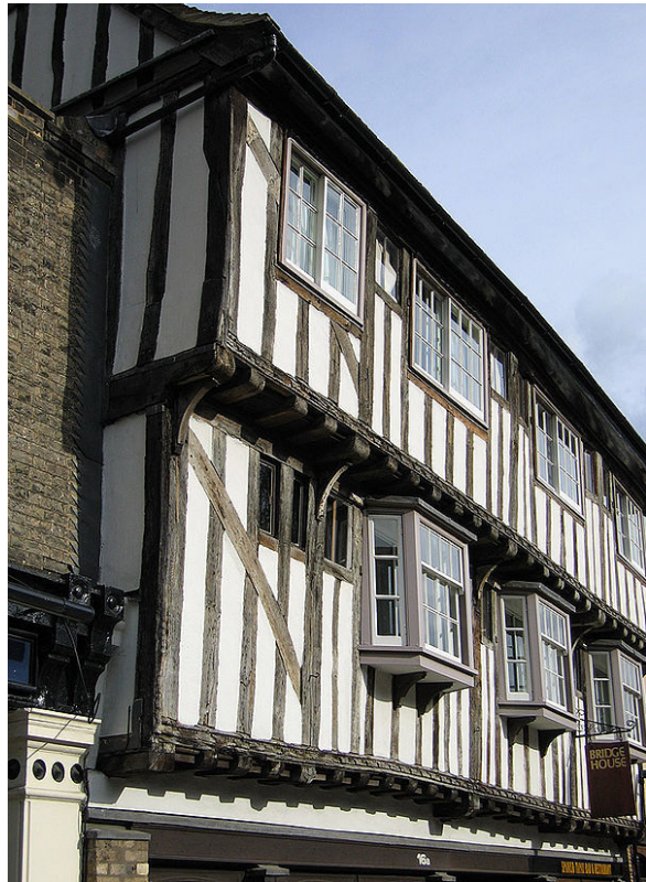
Projecting (“jettied”) upper storeys of an English half-timbered village terraced house, the jetties plainly visible
