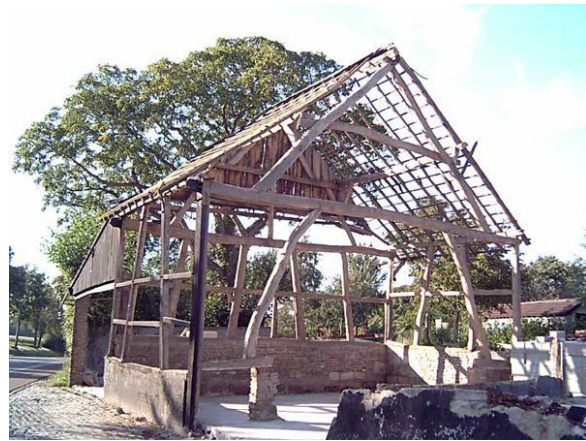
A half timbered building without the infill in Limburg, Netherlands.
