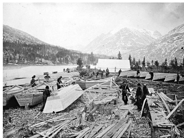
Wooden boats being built during the Klondike Gold Rush.
