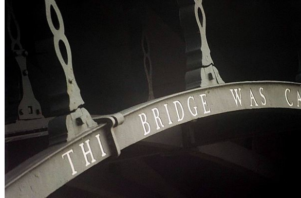
Cast iron dovetail joints in The Iron Bridge
