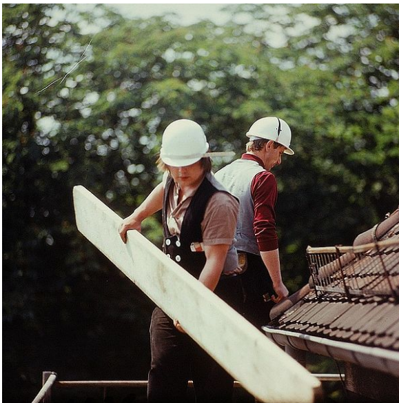
Two German carpenters working (1975)
