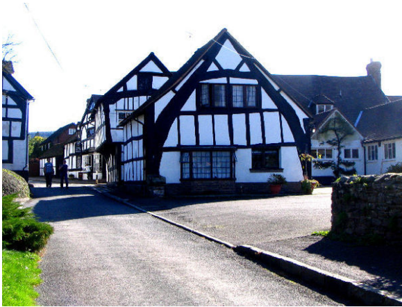
A “true” or “full” cruck half-timbered building in Weobley (Herefordshire, England). The cruck blades are the tall, curved timbers which extend from near the ground to the ridge.
