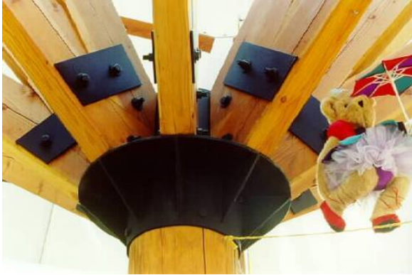
Metal plates are often incorporated into the design where the timber alone would not be strong enough for a given load.
