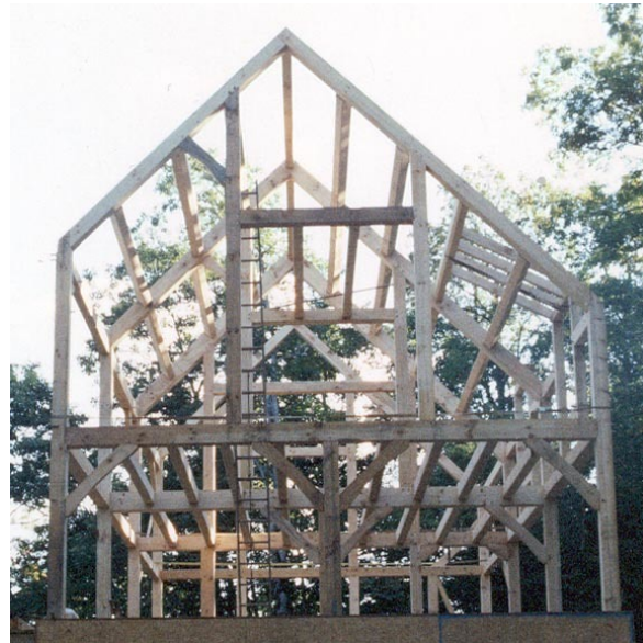
The completed frame of a modern timber-frame house
