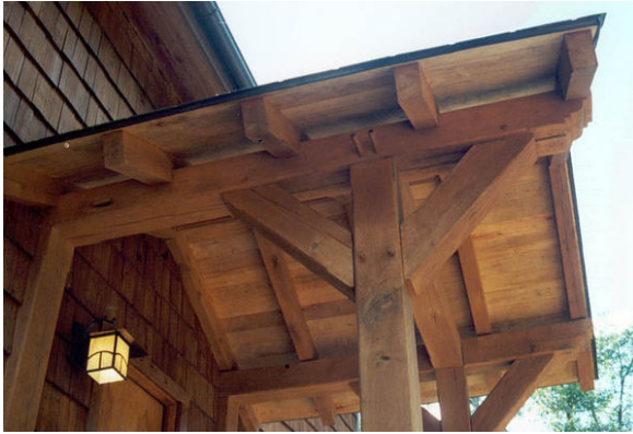
Porch of a modern timber-framed house
